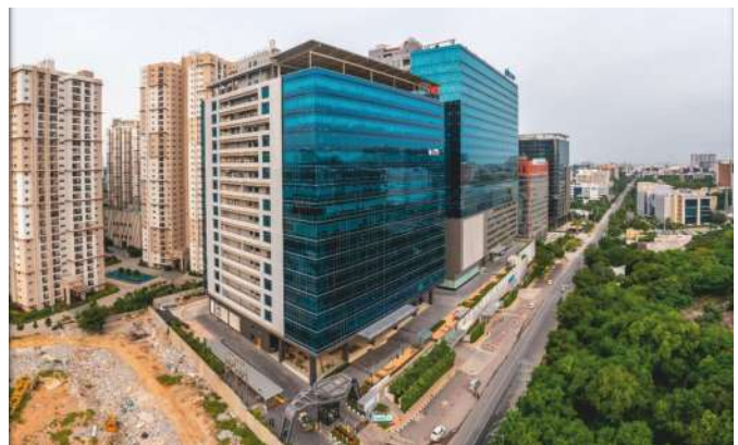
Image 1: Phoenix Aquila, Hyderabad (2 Basements + Ground Floor + 7 Stilt Floors + 16 Upper Floors.); Height:106 mtr; Area Apx: 1.3 Million sq ft ; Project Status: Structure Completed.
